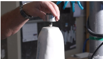
Put CD103FD fabrication dummy over anchor.
